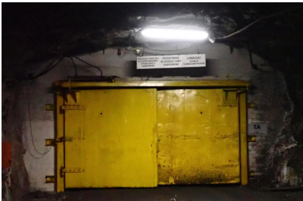
Figure 6.3. Example of ventilation lock used in KGHM mines
